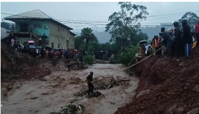
Place in Bamenda where a temporary foot bridge collapsed after water surge, killing at least 4 people, more likely 16.
