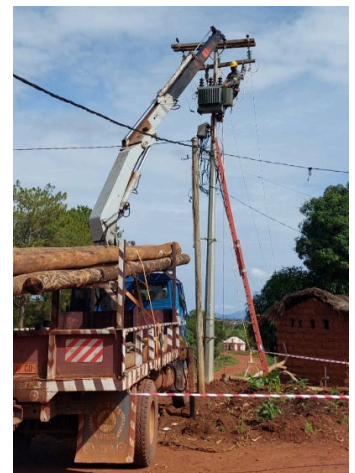
This equipment had to come from Ngoundere – about 12 hours away.
