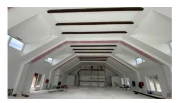
Work on the main lodge continues, with the goal of completing the second-floor dining hall and bathrooms before camps begin this summer. This past month, the crew has plastered the walls, leveled the cement floor, roughed in the bathrooms, and installed wood beams. The space continues to amaze us with how spacious and beautiful it is—we can't wait to fill it with campers again! Seeing the Farm to Field team's help finishing the exterior makes us excited to see the interior coming together, too.
