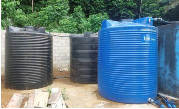
New water tanks
