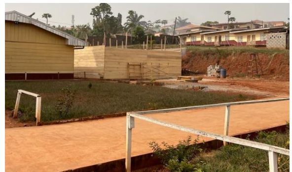
Maternity project under construction
