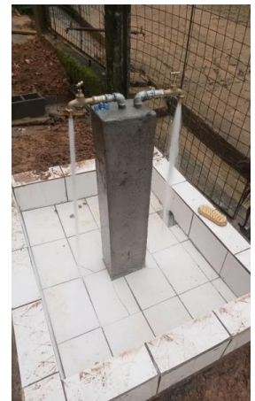
New water-collection point
